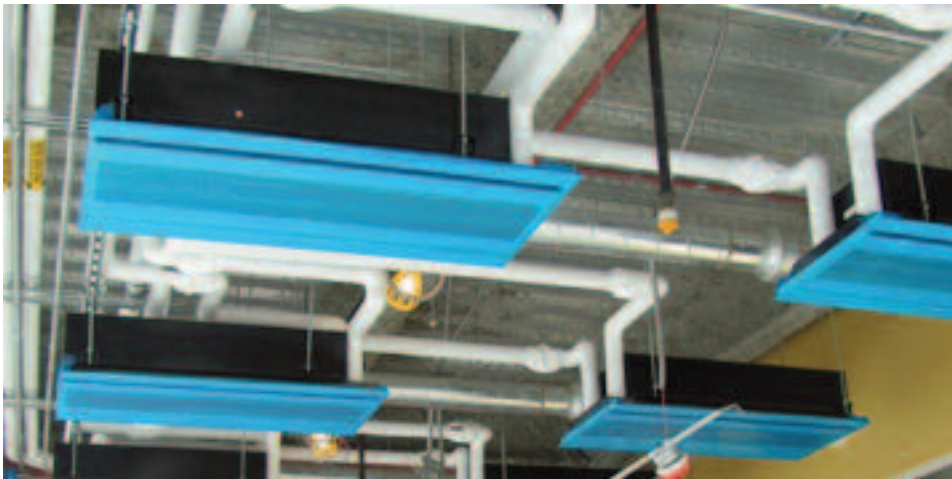
Active chilled beams with 1-way flow installed for lab application
